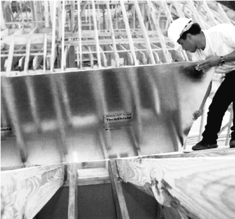
Figure 12.7 Radiant barrier laminate. (Louisiana-Pacific Corp., Tech-Shield)
